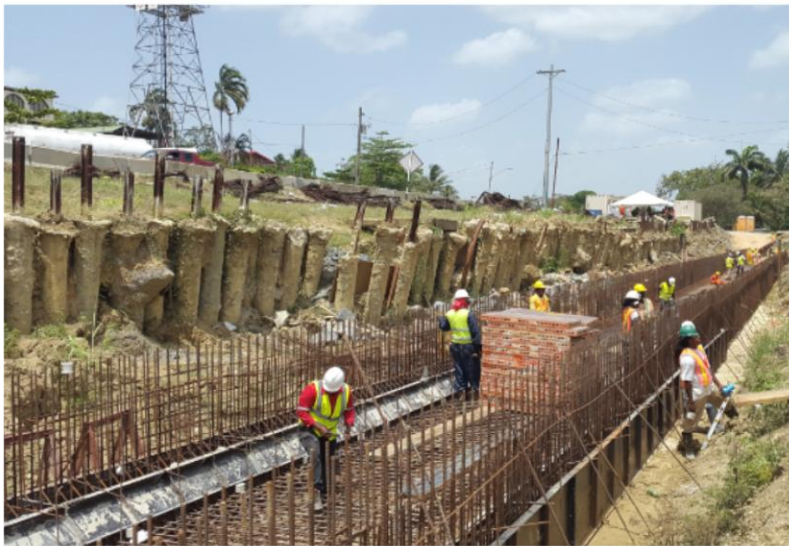
Sir Solomon Hochoy Highway Extension to Point Fortin – Construction of Reinforced open channel Retaining Walls 18
