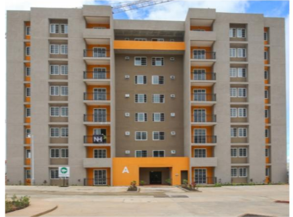
Residential Project: Mt Hope Apartments
