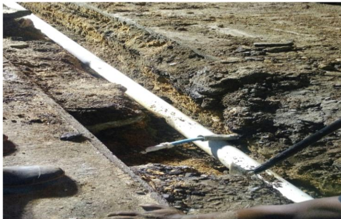
100mm Duct Construction – Chaguaramas to Westmoorings
